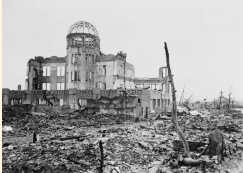
shutterstock_251930719.jpg Wrecked framework of the Museum of Science and Industry in Hiroshima, Japan. This is how it appeared shortly after the dropping of the first atomic bomb, on August 6, 1945.
